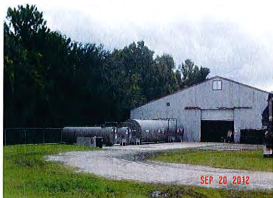
Photo 1 - area for tank expansion
