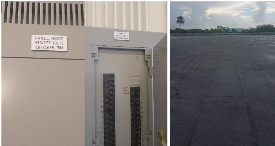
Tamarac Library Site Visit
