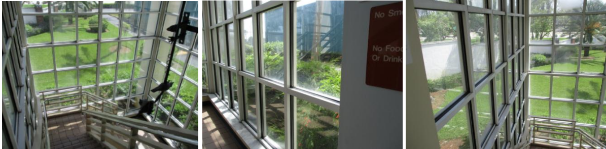
Interior view of area to receive film.
