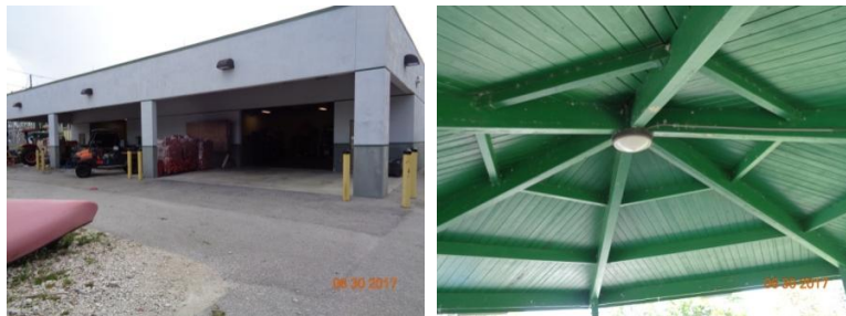
Exterior Lighting Examples
