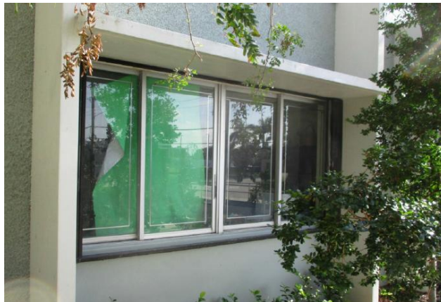
Occupants are attempting to keep heat out by use of paper and fabric
