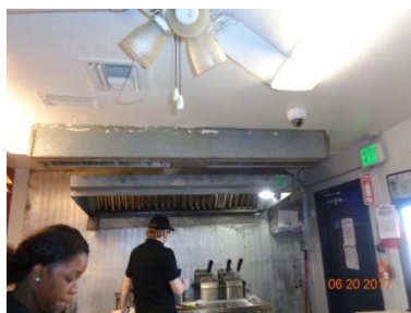
Interior Lighting Examples
