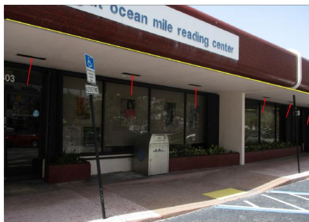
Large vents (red arrows) and strip vent (yellow line) shown here
