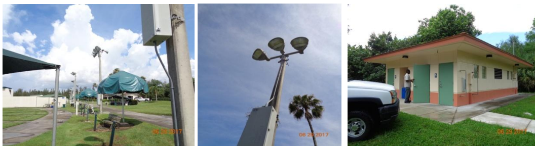
Exterior Lighting Examples
