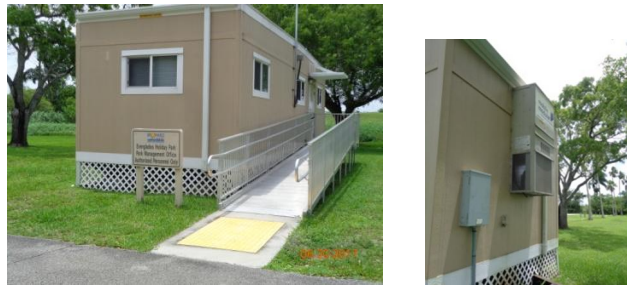
Camp Grounds Office HVAC
