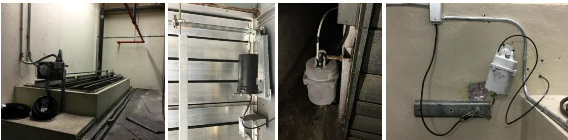
Return and Outside Air Damper Control
