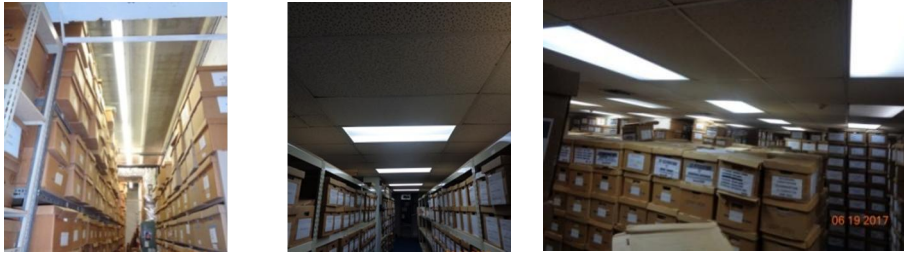
Interior Lighting Examples
