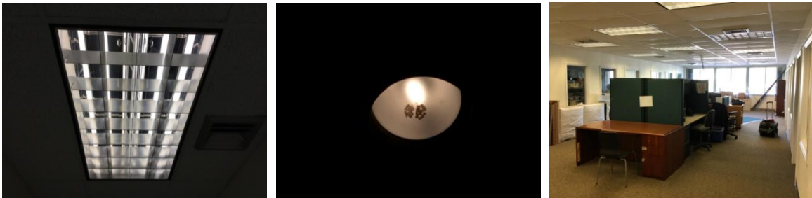
Interior Lighting Examples Pictured Above
