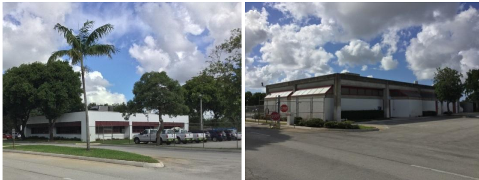
Highway and Bridge Facilities
