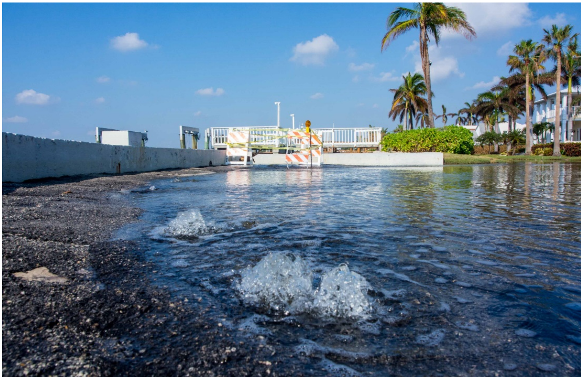
High tides can cause saltwater to flow up through porous asphalt
