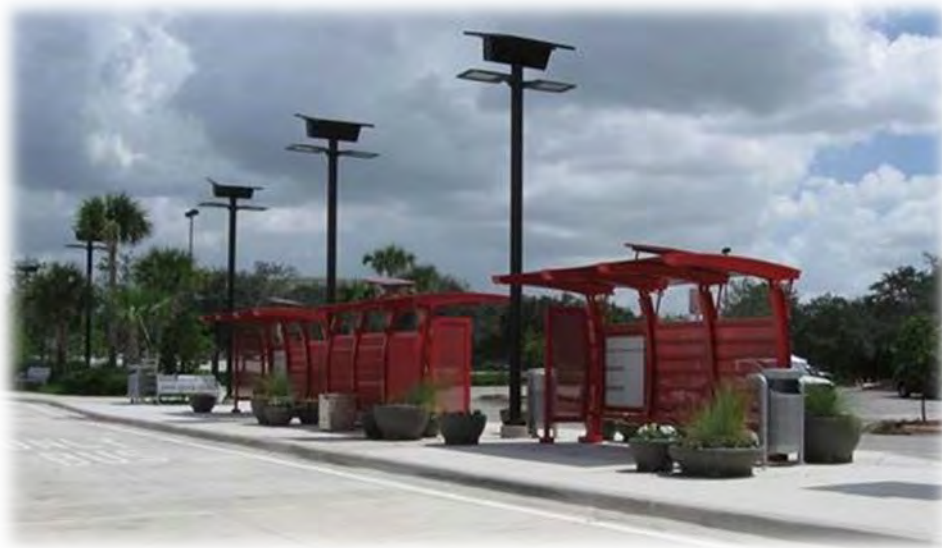
BB&T Center Park and Ride Lot for 95/595 Express Bus Service, an example of successful implementation of Policy T2.5.1
