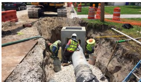
Drainage improvement project completed in Washington Park
