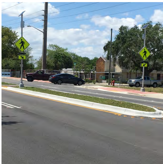
BMSD Safe Streets Project – Phase I : landscaped medians, decorative crosswalks with flashing beacon and bike lanes from NW 24 Ave and 6 Street (Sistrunk Blvd) – pictured- down to 27 Avenue
