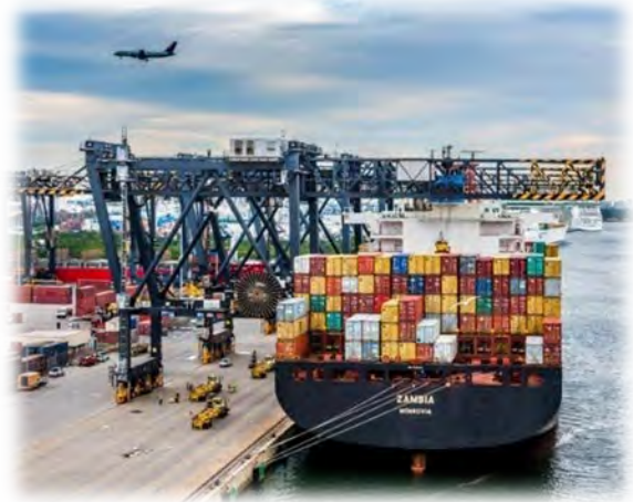
Port Everglades gantry crane
