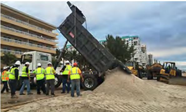
**Beach renourishment is a means of shore protection designed to retain and rebuild natural systems, such as beaches, while reducing or preventing the consequences of beach erosion.**
