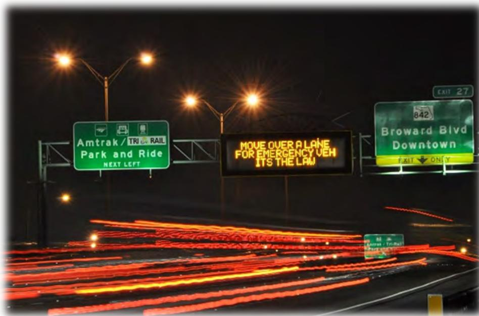
**Dynamic Message Signs (DMS) are a component of TSM&O (Policy 4.5.5) used to communicate travel times, crash and incident data, safety announcements, and AMBER/Sliver Alerts to the traveling public.**
