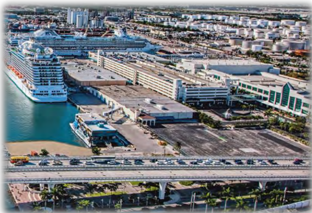
Aerial view of Port Everglades North Port
