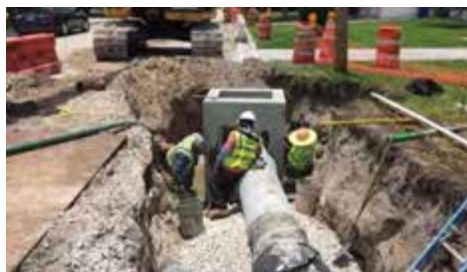
Drainage improvement project completed in Washington Park
