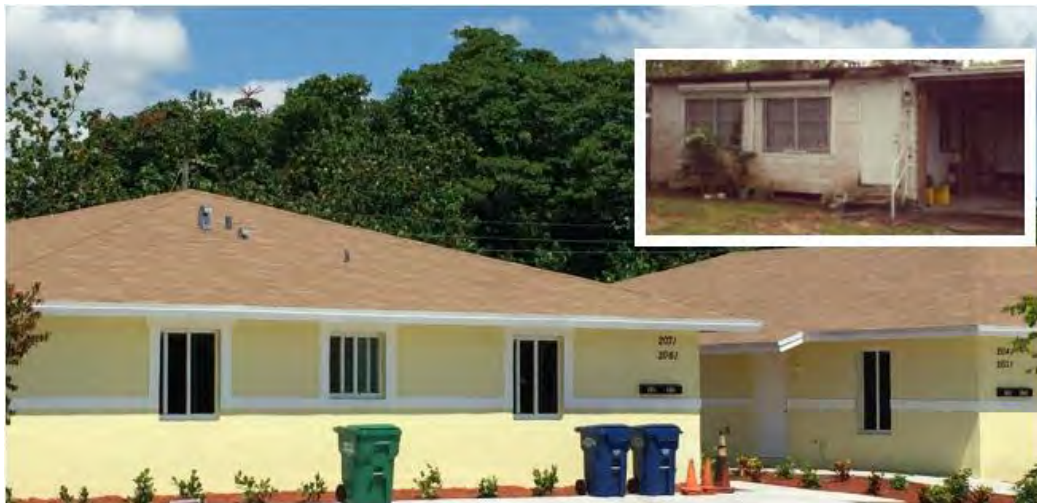
Code Enforcement influenced legal renovation of blighted unsafe structure into attractive occupied multi-family residence
