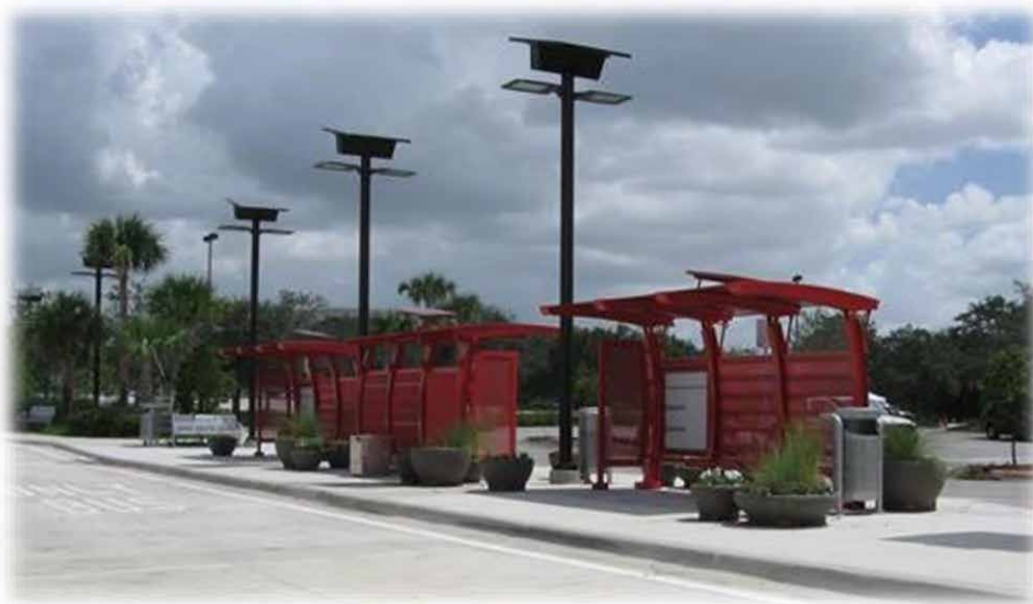
BB&T Center Park and Ride Lot for 95/595 Express Bus Service, an example of successful implementation of Policy T2.5.1
