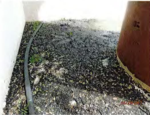
northwest corner of containment structure
