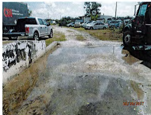
truck park area
