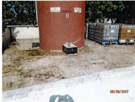
tank containment structure
