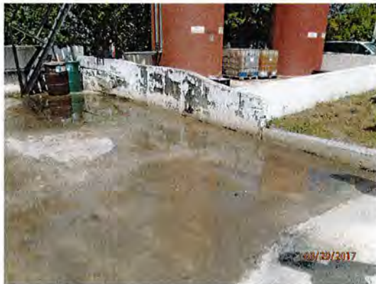
truck park area
