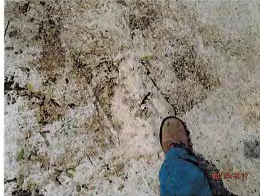
cracked/peeling sealant in containment structure
