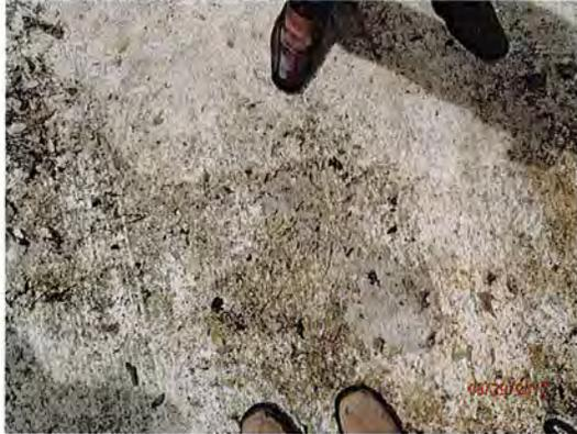
cracked/peeling sealant in containment structure
