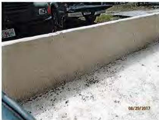
cracked/peeling sealant in containment structure
