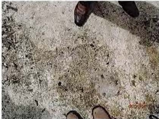
cracked/peeling sealant in containment structure
