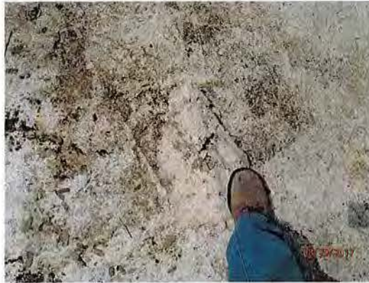
cracked/peeling sealant in containment structure
