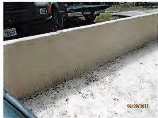
cracked/peeling sealant in containment structure
