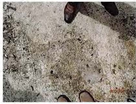
cracked/peeling sealant in containment structure
