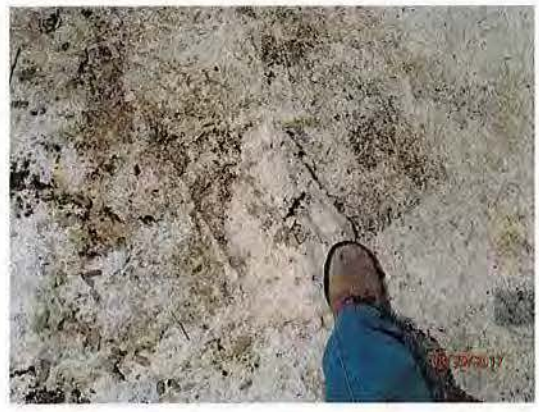
cracked/peeling sealant in containment structure
