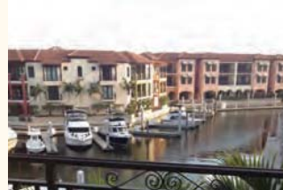
Example of three-story residential buildings embracing the adjacent canal in Naples.
