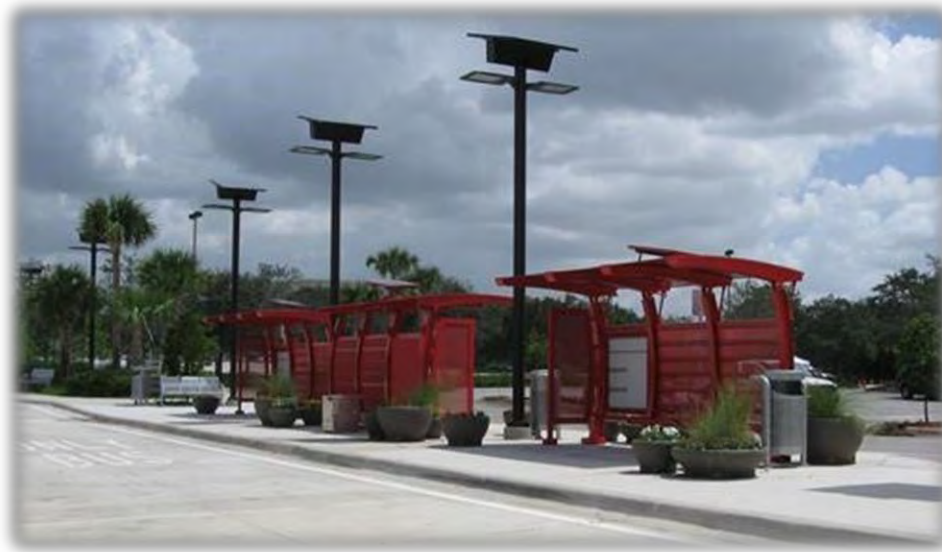
BCT BB&T Center Park and Ride Lot for 95/595 Express Bus Service, an example of successful implementation of Policy T2.5.1
