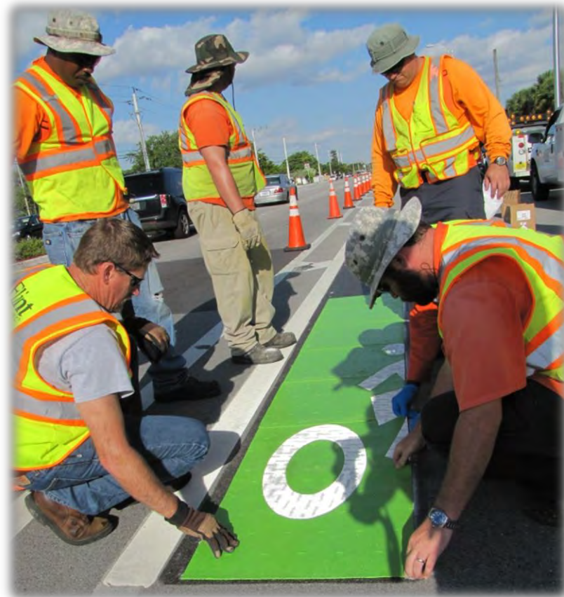
Installation of a green bicycle lane on Bailey Road, another Broward Complete Streets project.
