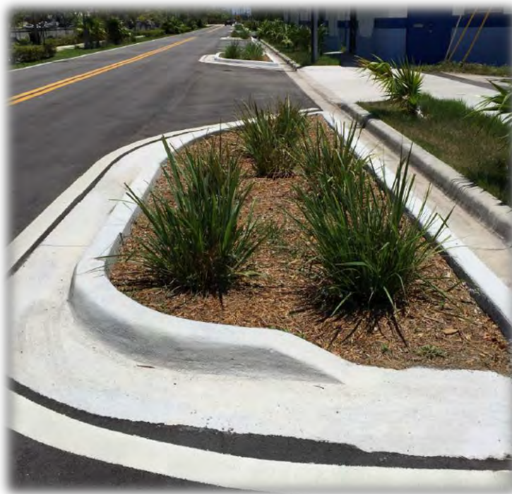
Flagler Drive Bioswale, Fort Lauderdale. Project that supports Policy T1.1.9.
