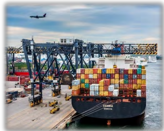
Port Everglades gantry crane
