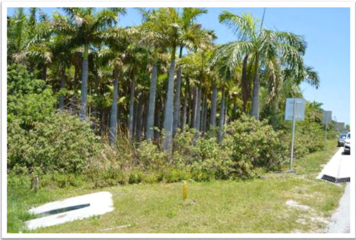
View of culvert along NE 10 th Street frontage
