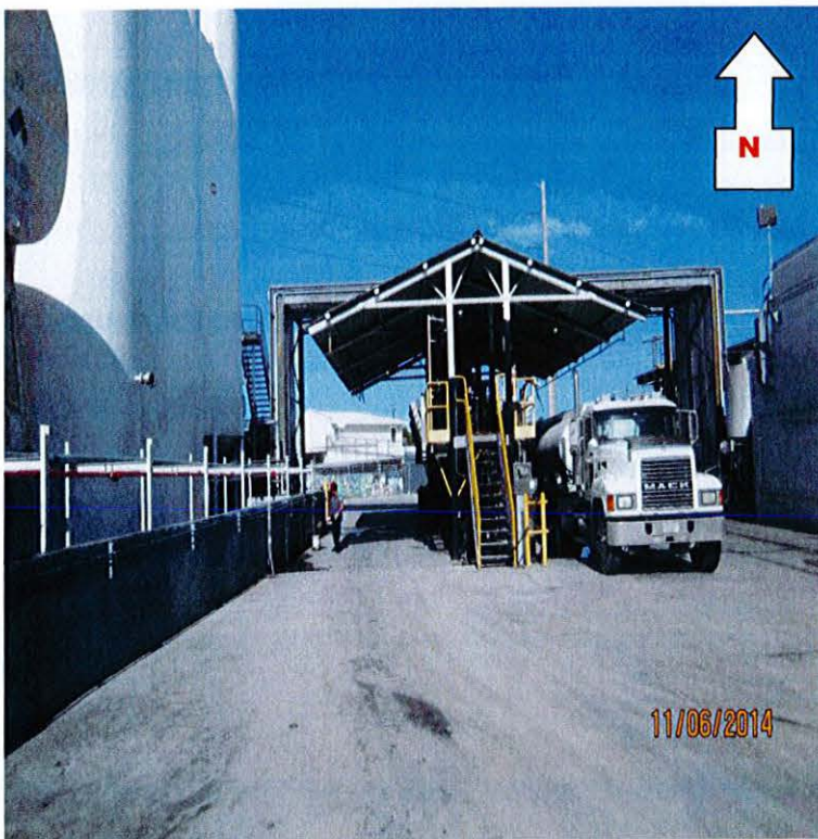
Mild, inconsistent odors were detected in on/off-loading area. The exact source of the odors was not determined.
