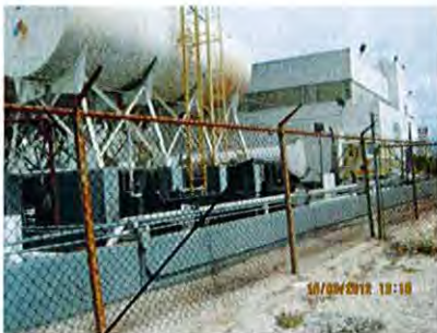
Truck off loading
