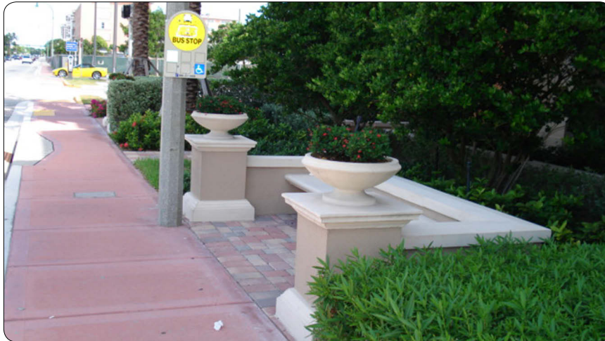
Figure 3.4.4 - Photo - Passenger Waiting Pad sidewalk.
