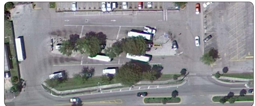
Figure 5.3.3 - Photo - Off-Street Facility - Aerial View-Lauderhill Mall Terminal
