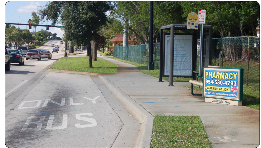
Figure 5.4.3 - Photo - Mid-Block Bus Bay
