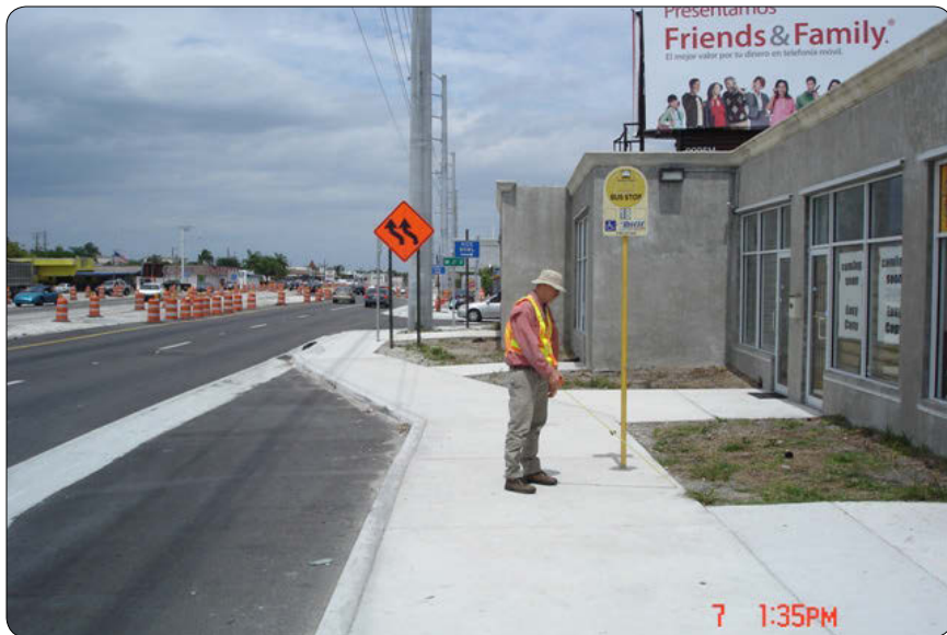
Figure 5.2.1 - Photo - Bus Bay and Sidewalk
