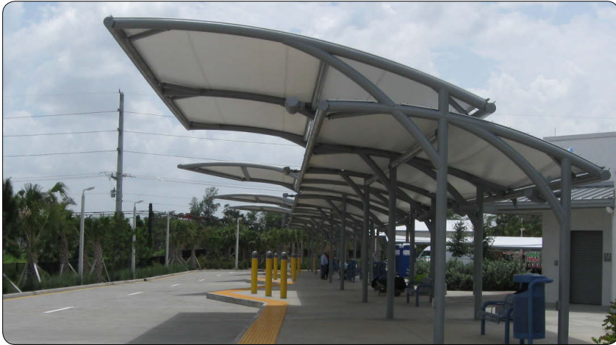
Figure 5.5.6 - Photo - Typical Bollard Placement at Bus Berth
