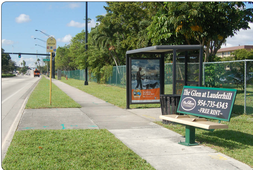
Figure 3.6.11 - Photo - Bus Shelter with Advertisement Panel
