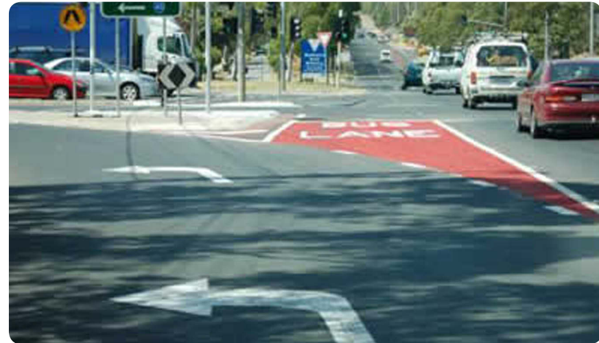
Figure 5.4.8 - Photo - Queue Jumper Bus Lane
