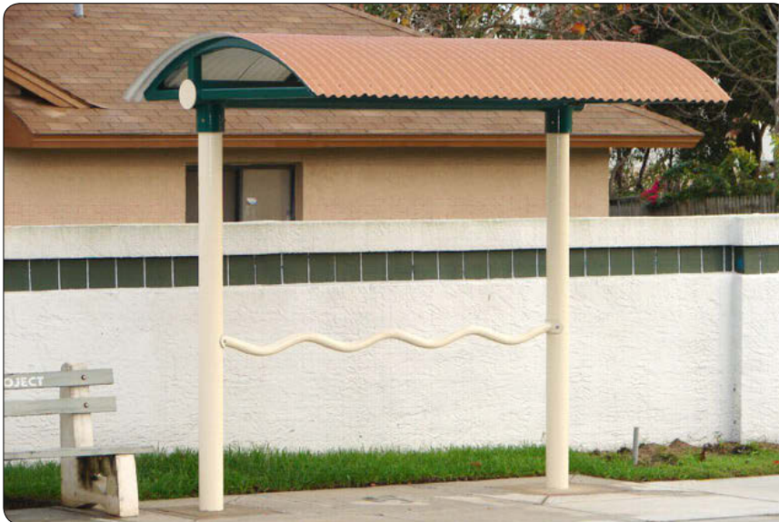
Figure 3.8.6 - Photo - Leaning Rail
