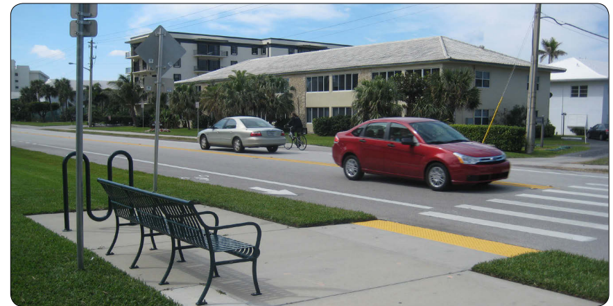
Figure 4.1.8a - Photo - Detectable warning strip at bus stop with no curb.
