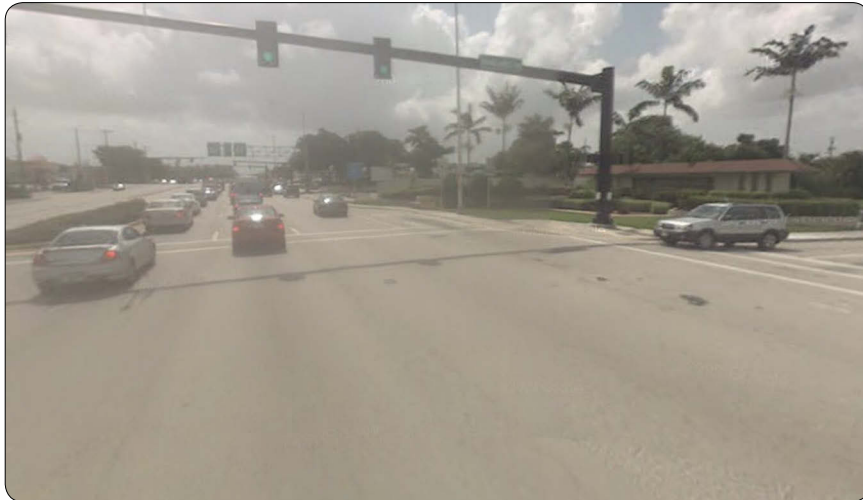
Figure 5.4.4 - Photo - Open Bus Bay
