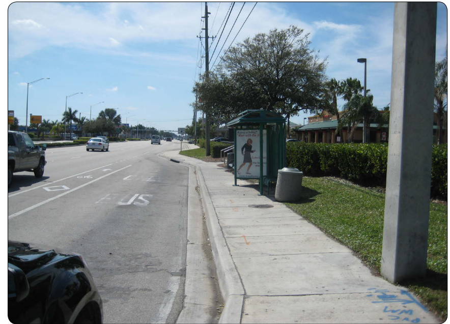
Figure 5.4.1 - Photo - Typical Bus Bay
