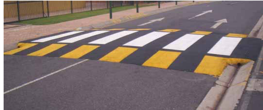
Figure 5.2.19 - Photo - Speed Bump
