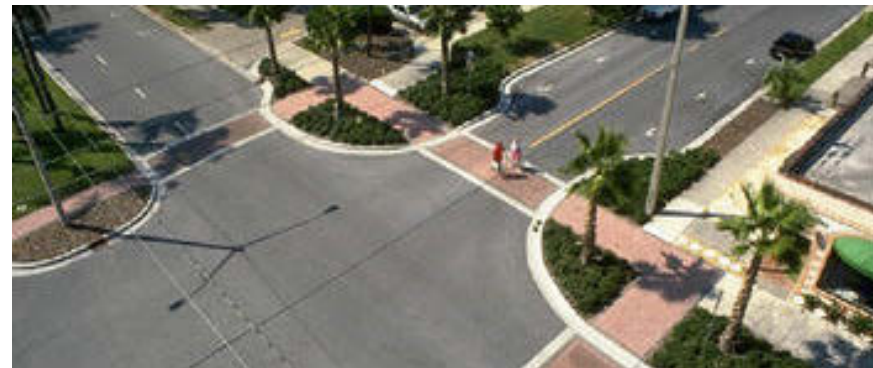
Figure 5.2.20 - Photo - Choke Point (Bulb Outs)
