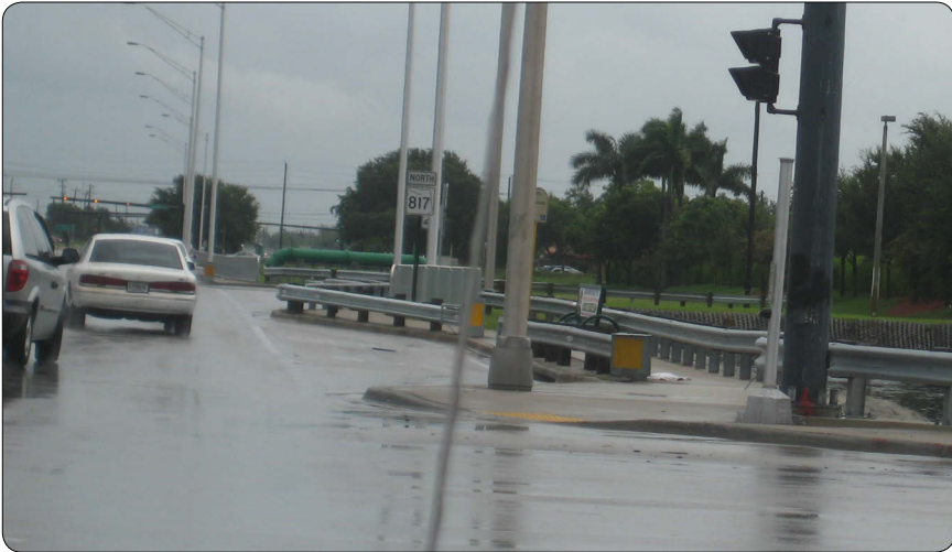
Figure 5.4.6 - Photo - Partial Open Bus Bay
