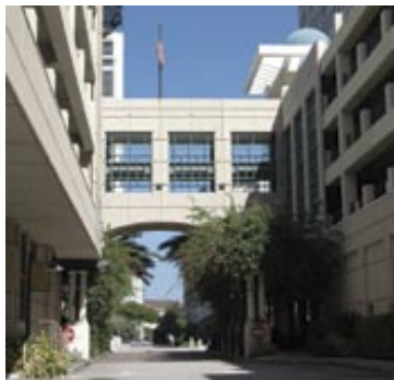
Indoor parking structures connected by an open walkway bridging across the street encourages air-circulation and creates a pleasant breezeway access to Las Olas Boulevard.
