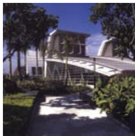
Landscaping provides shade on a walk leading to a transit station in Hong Kong.
