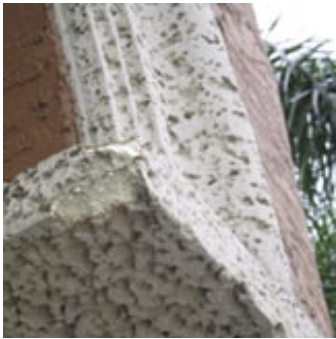
Details are important at the slow pace and scale of the pedestrian. The use of polystyrene plastic foam in places where people come into contact with buildings promotes a false impression and does not hold up well.
