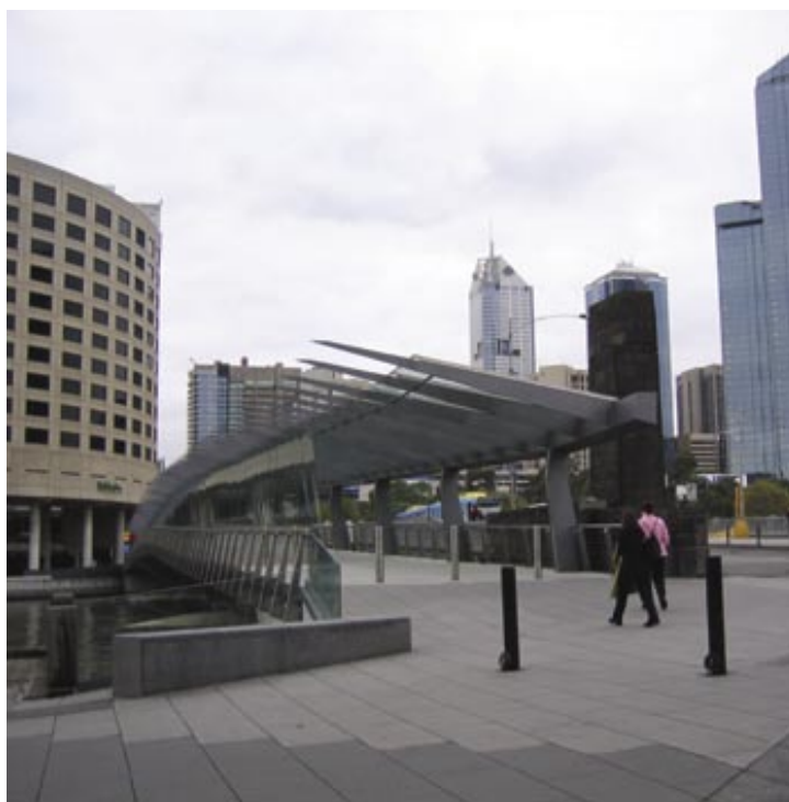
A glazed canopy and wall provide weather protection on a bridge with unimpeded pedestrian and bicycle access across the Yarra River at Spencer Street in Melbourne, Australia.
