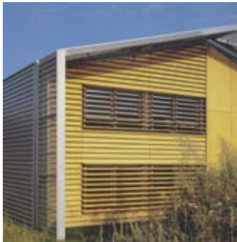
Effective use of louvers, grills, and screens, and overhangs provide a transition from indoor to outdoor light.
