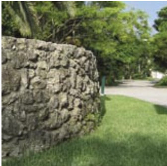
Native oolitic limestone is used on this site wall, capturing a sense of place.
