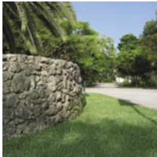
A natural stone wall of local oolitic limestone is an example of a material selection that reinforces our sense of place.
